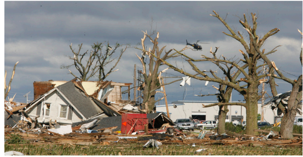
The aftermath of a devastating tornado that struck the Toledo area on June 5, 2010. Photo courtesy of The Toledo Blade
